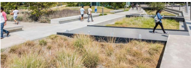
Stormwater infiltration basins should be integrated throughout the design to reduce off-site detention needs and improve water quality.
